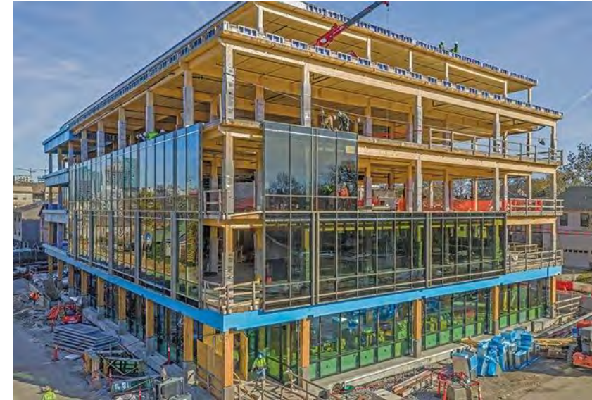
Mass timber construction
