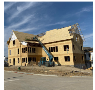
Figure 2.4 The simple forms, smaller size, and compatibility with simple wood-frame construction help maximize affordability and investment returns, and are consistent with the construction strategies familiar to most residential homebuilders, as shown in this under-construction MMH project in Papillion, Nebraska.
