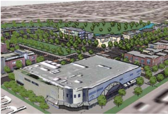
Development at the corner of North Wolf Road and North Avenue will serve as a focal point for a mixed-use, walkable neighborhood.
