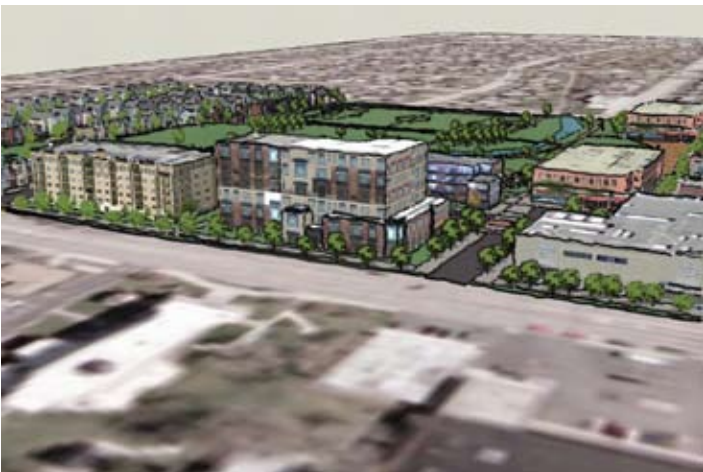
Mixed-use development along North Wolf Road will complement the new Wolf Ridge Condominiums.
