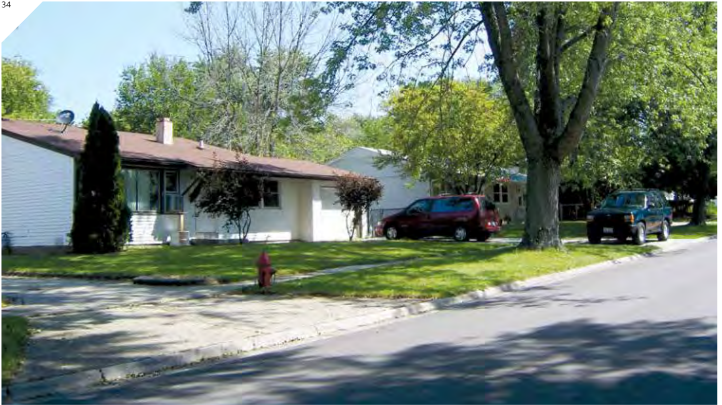
New residents could occupy currently vacant units.
