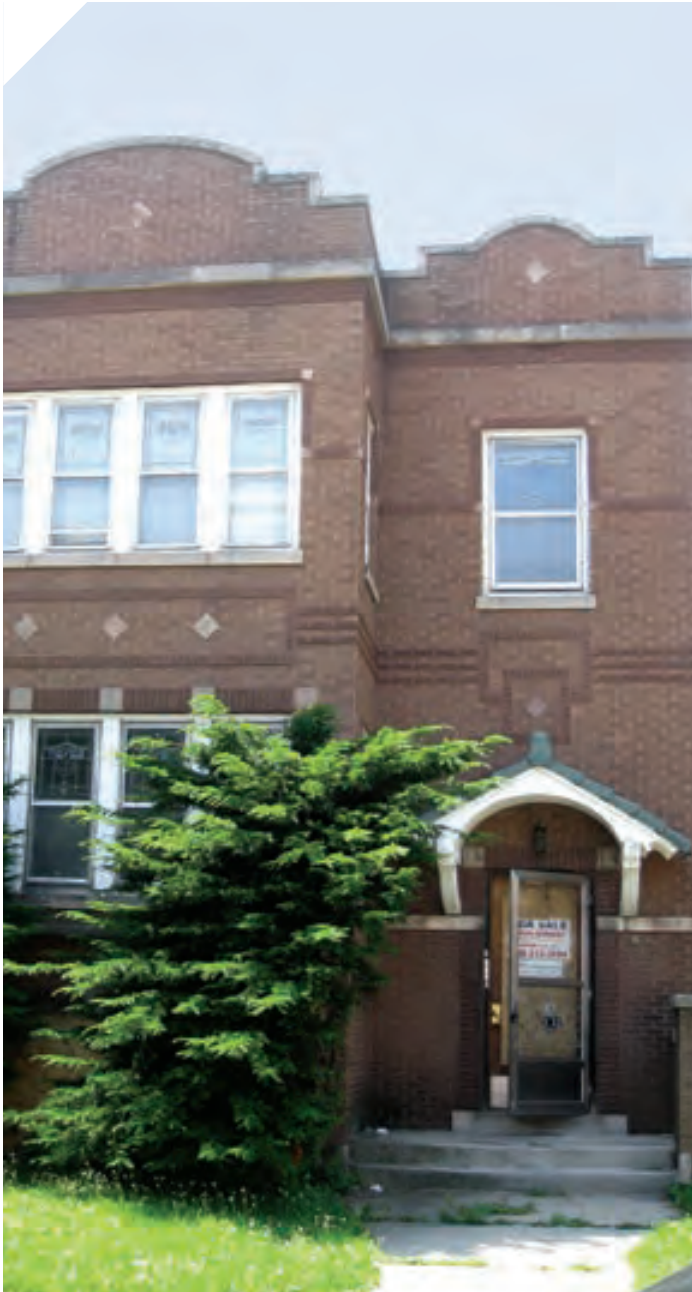
Foreclosure filings have increased especially in small multifamily buildings.
