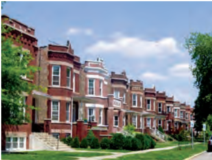
Like many older municipalities in the region, Berwyn has a substantial stock of 2- and 3-flat brick walk up buildings.
