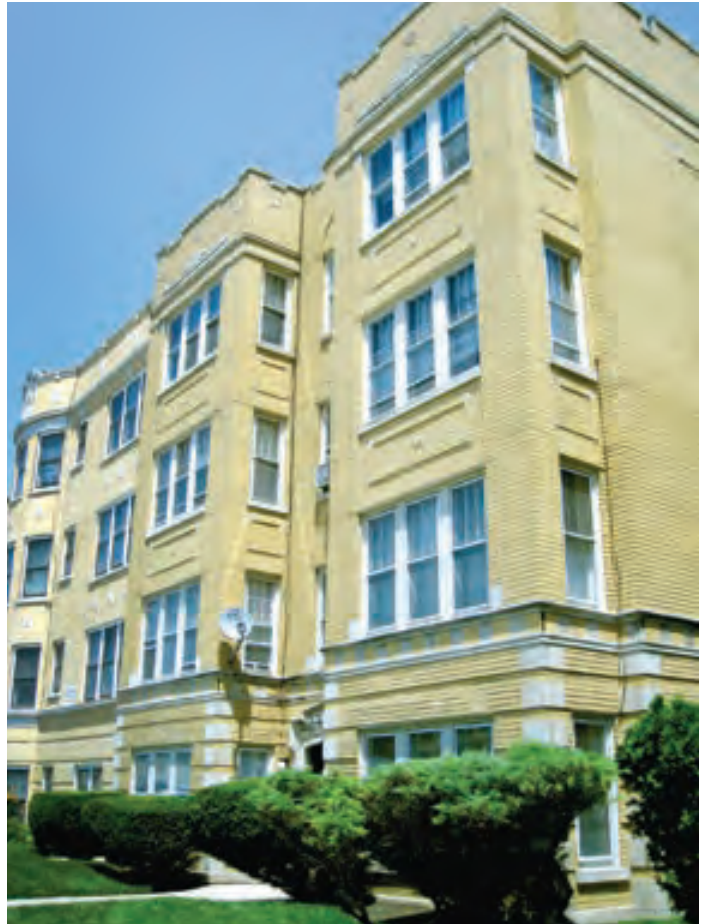
Multifamily buildings in Berwyn range from 2- and 3-flats to larger buildings like this one.
