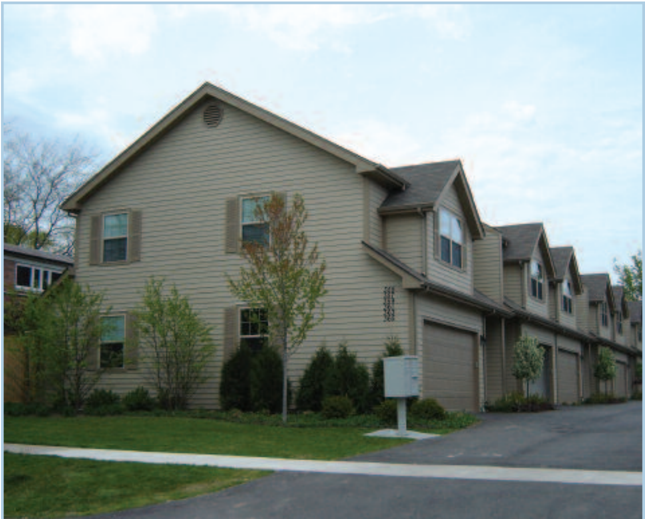
The Highland Park Illinois Community Land Trust owns these six affordable town homes in Highland Park. In this community, where the median home value is almost $430,000, these town homes sold for no more than $140,000.
