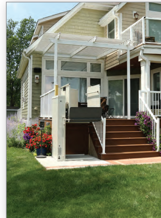
Above: A Vertical Platform Lift (VPL) added to an existing porch
