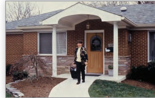
Above: An example of a renovated graded entry.
