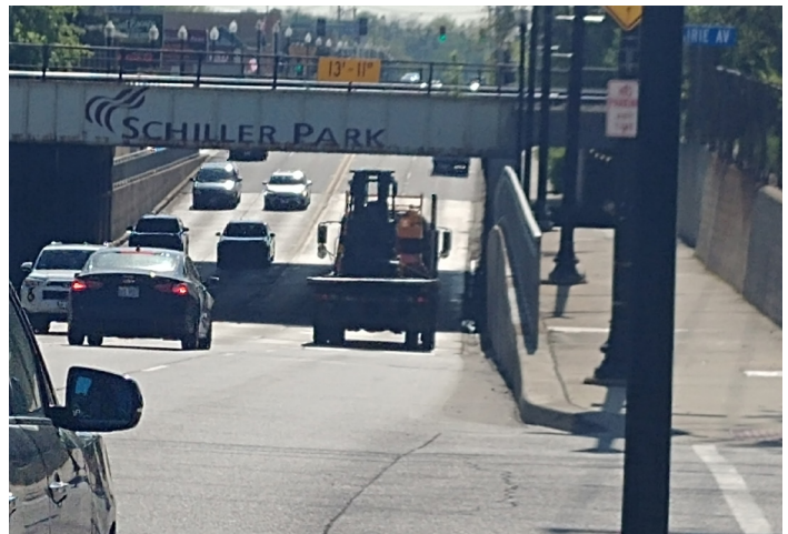
The very prominent underpass at Irving Park Road
