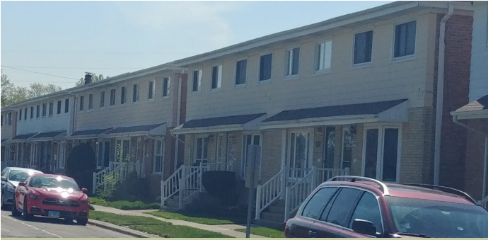
Townhomes along Soreng Avenue and Garden Court
