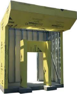
Location: Main entrance and roof
