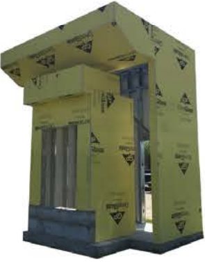
Location: Bay window bump out and roof condition
