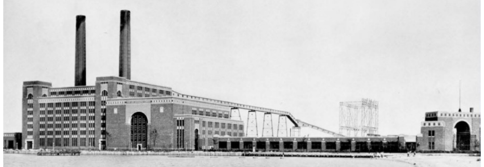
Stateline Power Plant (Hammond, Indiana) connected to the local ComEd distribution system
