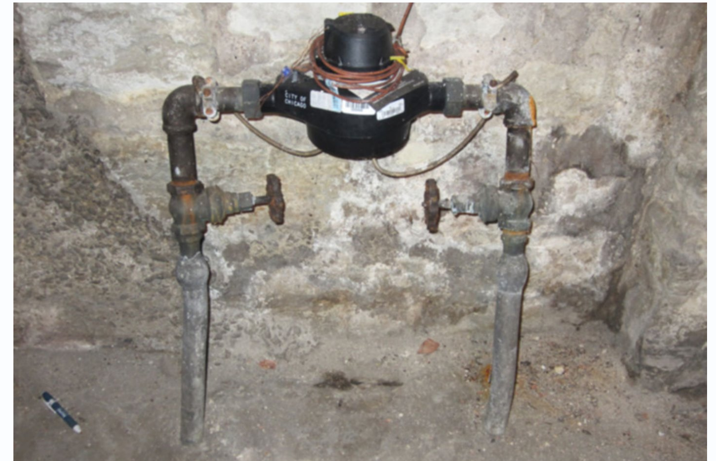
Residential Lead Service Line Connected to Water Meter
