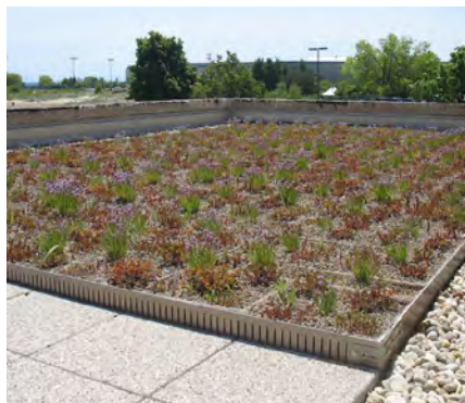
+ New solar panels (left) and green roof (right) on Evanston's Water Treatment Plant (Images courtesy of the City of Evanston)
